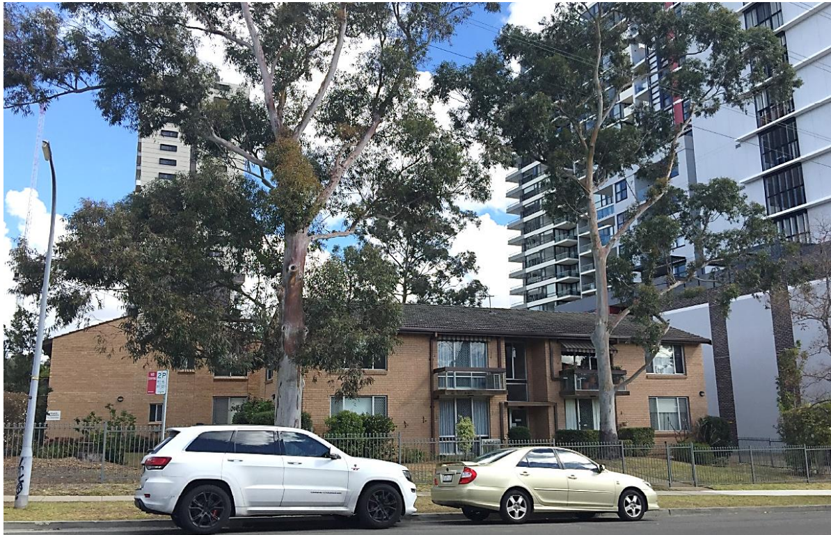
Figure 3. Site as viewed from Chester Street looking south.
